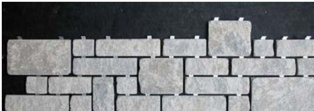
**Figure 2. "Shouldice Fusion Stone" installed for the Grouted Joint Design Just Before Grouted**
